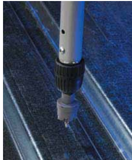
Drill Deck Holes
