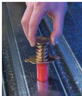
Push Anchor into Place
